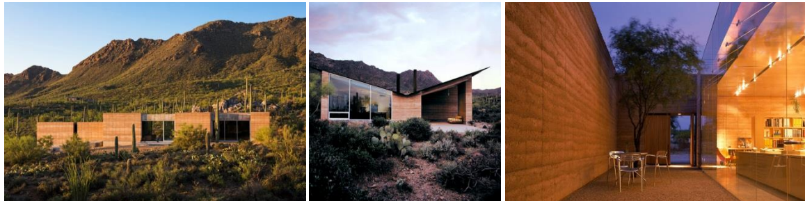
Fig. 30 : Rick Joy: Tucson Mountain Retreat ; Tucson Mountain House ; Rick Joy Architecture Studio (Sources : http://www.finehomebuilding.com ; http://www.rickjoy.com/ )
